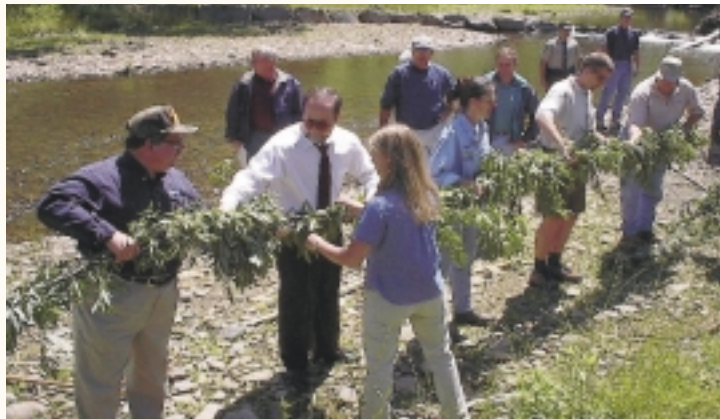
Volunteers from the Kettle Creek Watershed Association learn how to restore Kettle Creek using natural stream design methods. They are planting willow bundles that will help stabilize the stream bank when they sprout. Volunteers included Secretary of Environmental Protection David Hess, Kettle Creek Watershed Director Amy Gottesfeld, representatives from the offices of U.S. Rep. John Peterson and state Sen. Jake Corman, the Fish and Boat Commission, the Clinton and Potter County Conservation Districts, the U.S. Fish and Wildlife Service, and Dominion Transmission.
