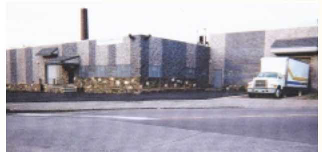
After, the newly renovated and updated building houses Custom Co-Pak, a tea-packaging company located in the heart of Philadelphia's Keystone Opportunity Zone. At this site, Governor Schweiker announced that more than 10,000 new jobs have been created in KOZ's statewide, where local governments, school districts and the state eliminate taxes to stimulate job creation and renewal in some of the Commonwealth's most challenged communities.
