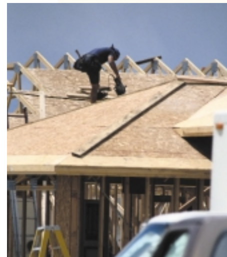
Another new home being built
